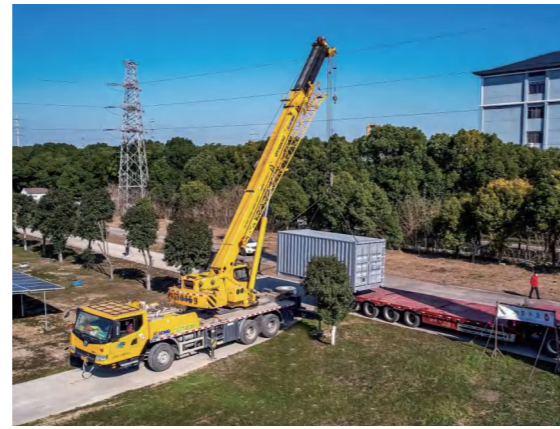
② Hoisting in Position
