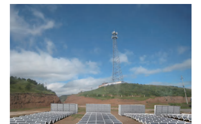
Telecom Tower Station
