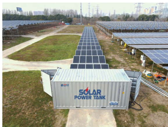
⑤ Cable Installation
