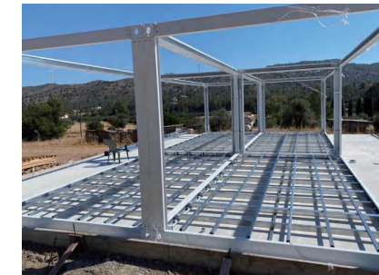
② 结构安装 Structural Installation
