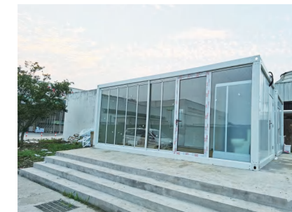
⑤ 安装门窗 Install doors and Windows
