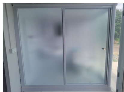
④ 安装一体式卫浴 Install Integrated Bathroom
