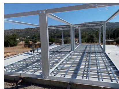
② 结构安装 Structural Installation
