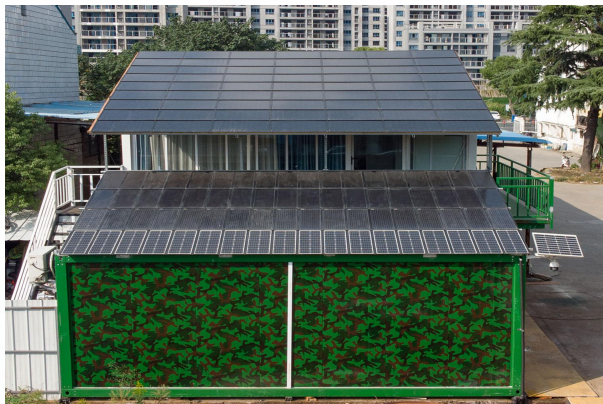
Solar PV system
