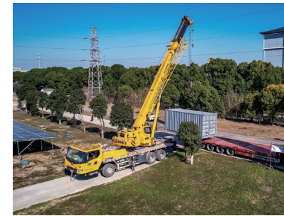
② Hoisting in Position
